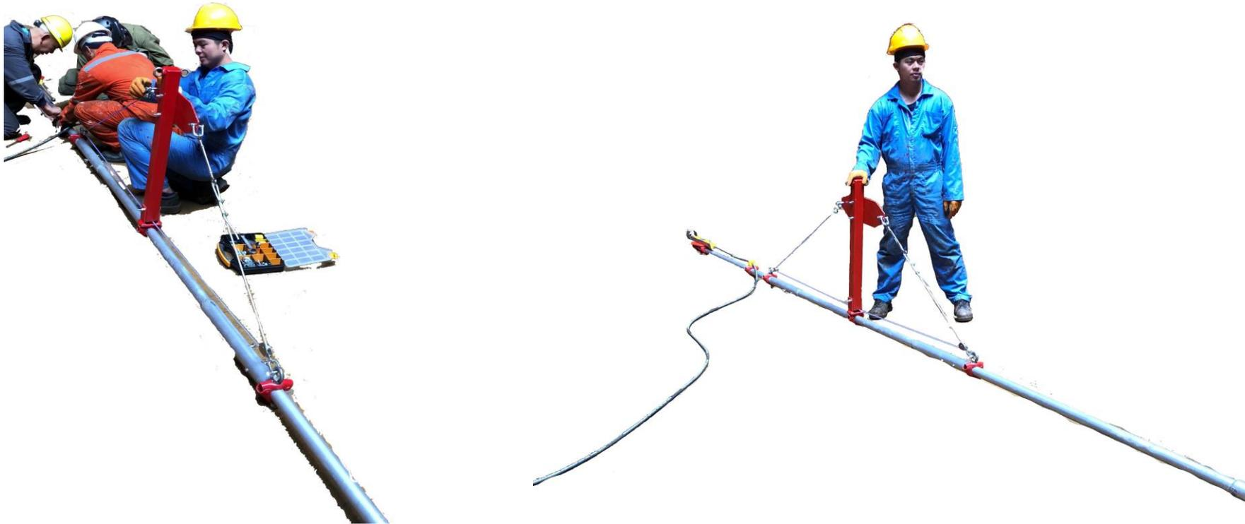
Complete the assembly with connecting the tension wire rope with fixed couplers, mini stainless steel pulley, clams, schakle and turnbuckle.
