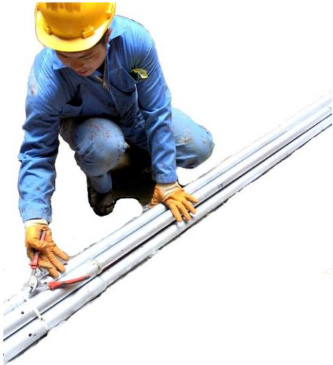
Expand the pipes to prepare the assembly.
