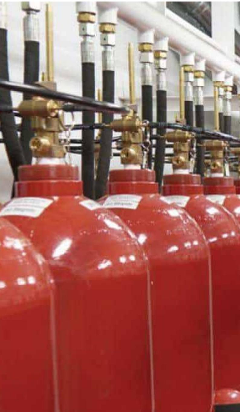
**1SN flexible rubber hoses reinforced by one steel wire braids complete with straight, 90 degree & swivel end fittings.**
